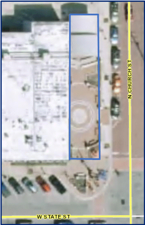
Spray Plaza Park Area
