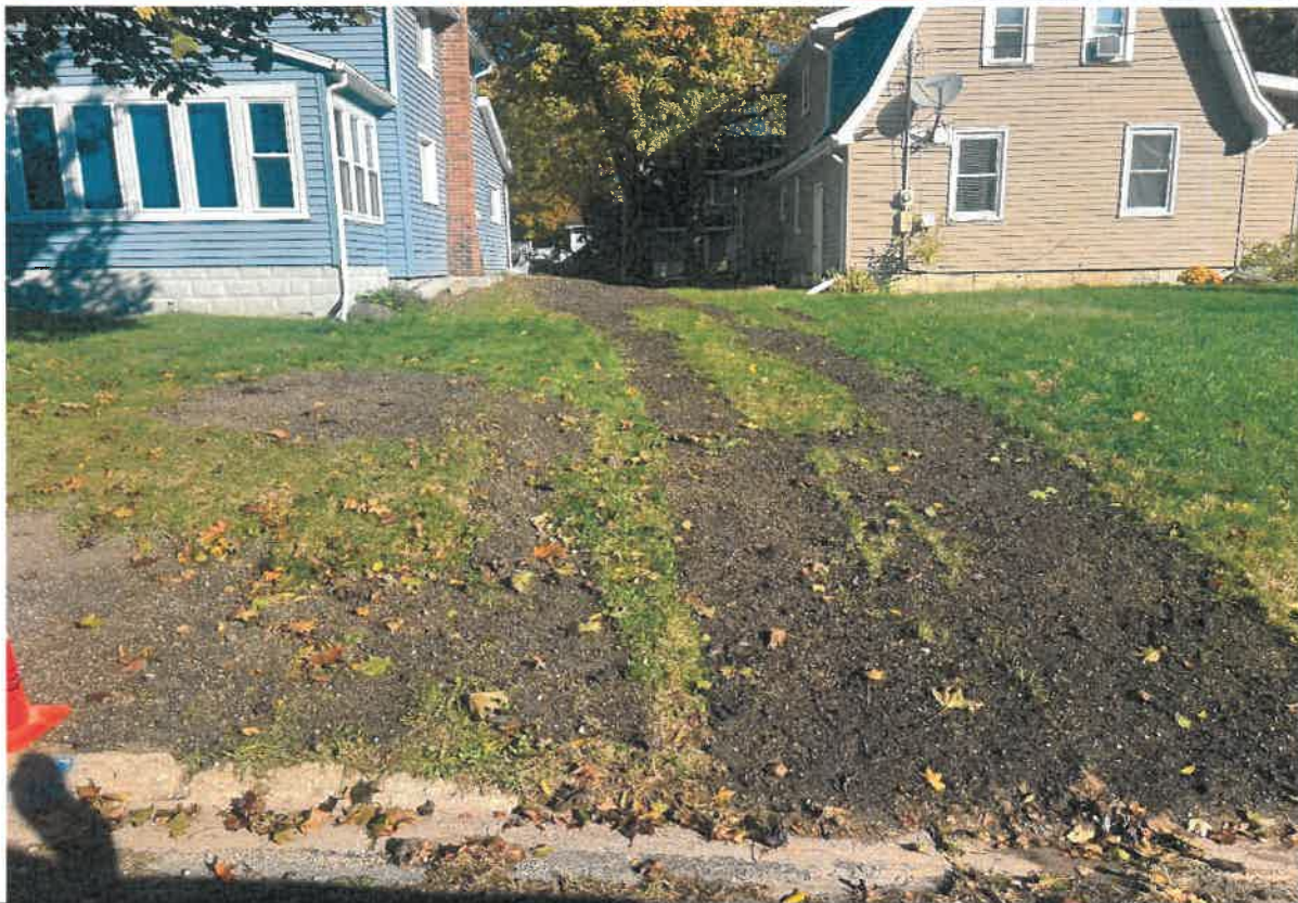
Occasionally DPS crew repairing lawns that were disturbed from the replacement program
