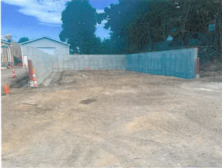
Figure 1 Salt Storage Shed walls and foundation
