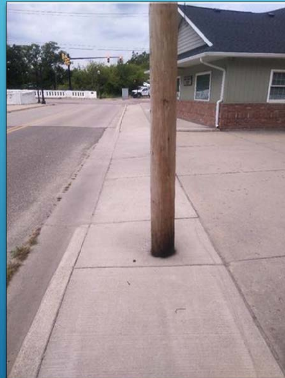
Telephone Pole Blocking Sidewalk in front of 201 East Mill St
