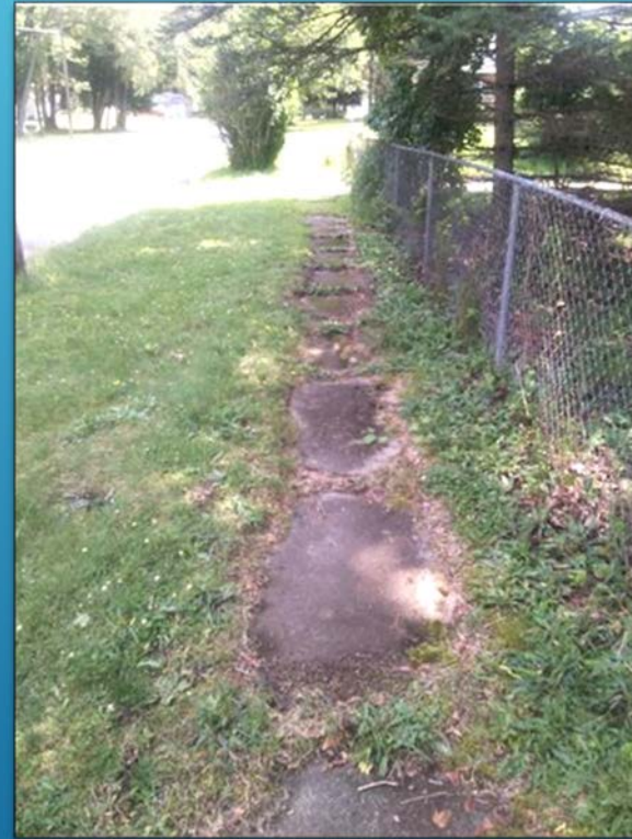
Grass and weeds overtaking the sidewalk in front of 610 East Thorn St
