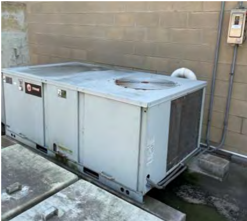
Figure 3-Make-up Air Unit
